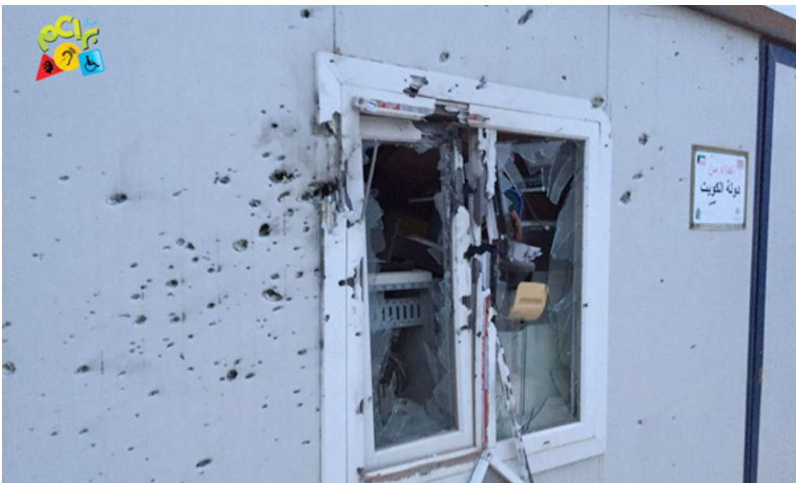
The aftermath of the Russian attack on Baraem Center. Source: Baraem Center.
